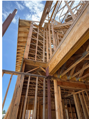
Front Entry Framing
